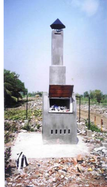
Incinerator for burning waste
